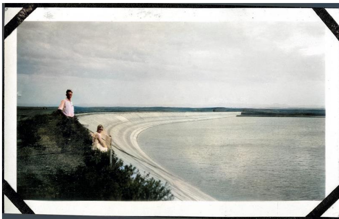
Belle Fourche Dam
