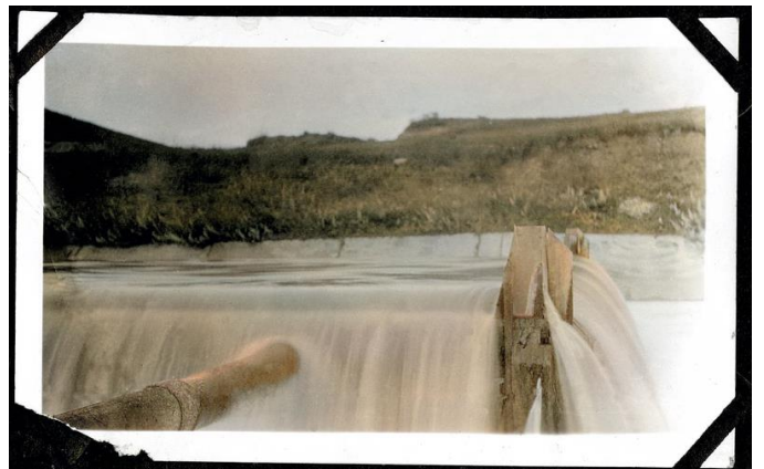
Overflow at Dam
